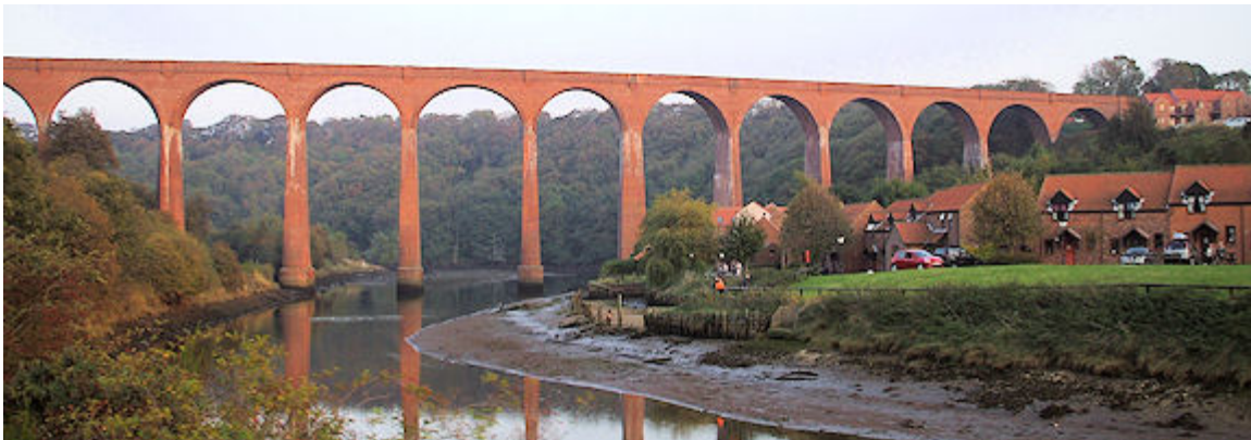
The Larpool viaduct on the outskirts of Whitby
